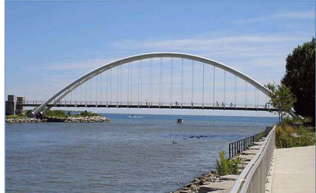
Steel Arch Bridge
