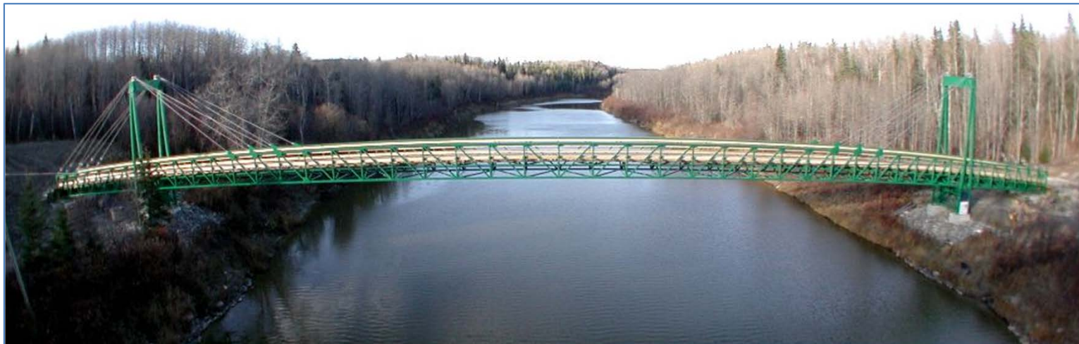
Steel Cable Bridge
