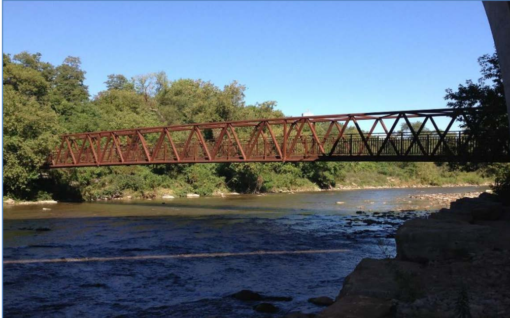
Steel Truss Bridge
