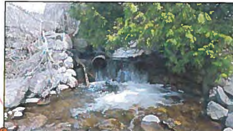
Feature #5: Fieldstone weir with clay pipes (listed, non-designated significant feature). No impact to feature anticipated. Feature is a substantial barrier to fish passage and limiting factor in overall channel function and health. Feature to be taken off-line/disconnected from active flow as a result of channel realignment. Feature will be maintained in landscape but will be impacted by loss of flow.
