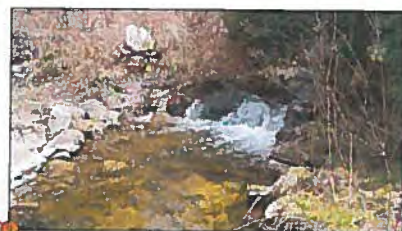
Feature #9: Fieldstone weir (listed, non-designated significant feature). No impact to feature anticipated. Feature is a substantial barrier to fish passage and limiting factor in overall channel function and health. Feature to be taken off-line as a result of channel realignment. Feature will be maintained in landscape but will be impacted by loss of flow
