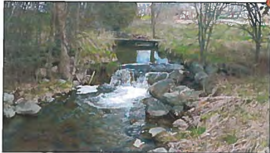
Feature #8: Fieldstone weir (listed, non-designated significant feature). No impact to feature anticipated. Feature is a substantial barrier to fish passage and limiting factor in overall channel function and health. Feature to be taken off-line/disconnected from active flow as a result of channel realignment. Feature will be maintained in landscape but will be impacted by loss of flow.
