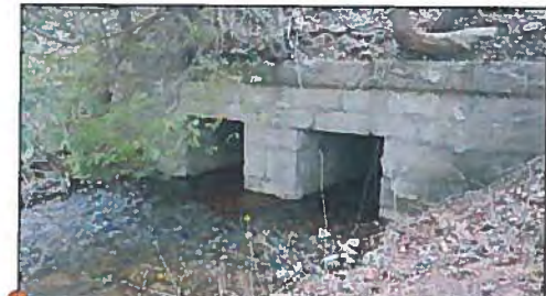
Feature #1: Aahar stone culvert (potential significance). No impact to feature anticipated.
