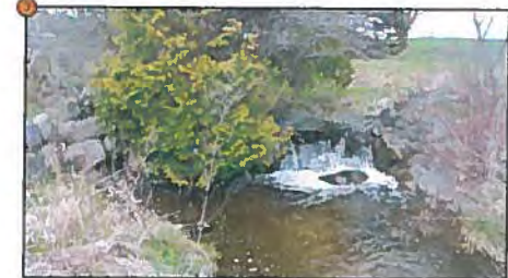
Feature #3: Fieldstone weir with steps and sentinel stones (listed, non-designated significant feature). Feature is a substantial barrier to fish passage and limiting factor in overall channel function and health. Feature to be taken off-line/disconnected from active flow as a result of channel realignment. Feature will be maintained in landscape but will be impacted by loss of flow.
