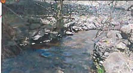
Feature #10: Fieldstone weir (listed, non-designated significant feature). No impact to feature anticipated. Feature is a substantial barrier to fish passage and limiting factor in overall channel function and health. Feature to be taken off-line/disconnected from active flow as a result of channel realignment. Feature will be maintained in landscape but will be impacted by loss of flow
