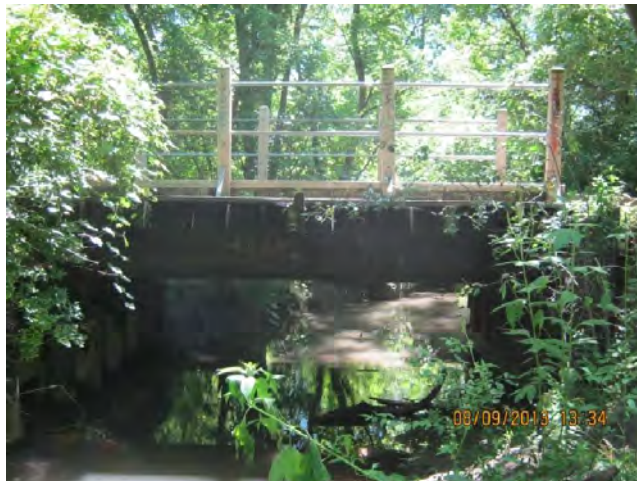
Figure 15: Typical steel girder bridge repurposed for pedestrian/cyclist use.
