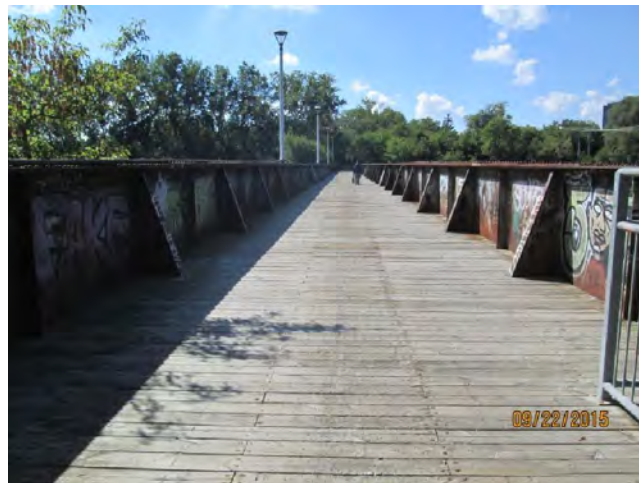
Figure 12: Through deck steel girder bridge (railway bridge repurposed for pedestrian use).
