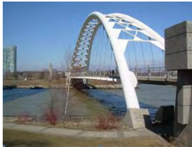
Figure 16: Humber River bicycle-pedestrian bridge (Source: Toronto and Region Conservation Authority).
