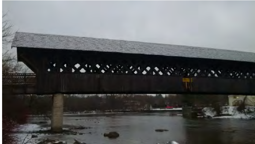
Figure 13: Covered bridge over Speed River.
