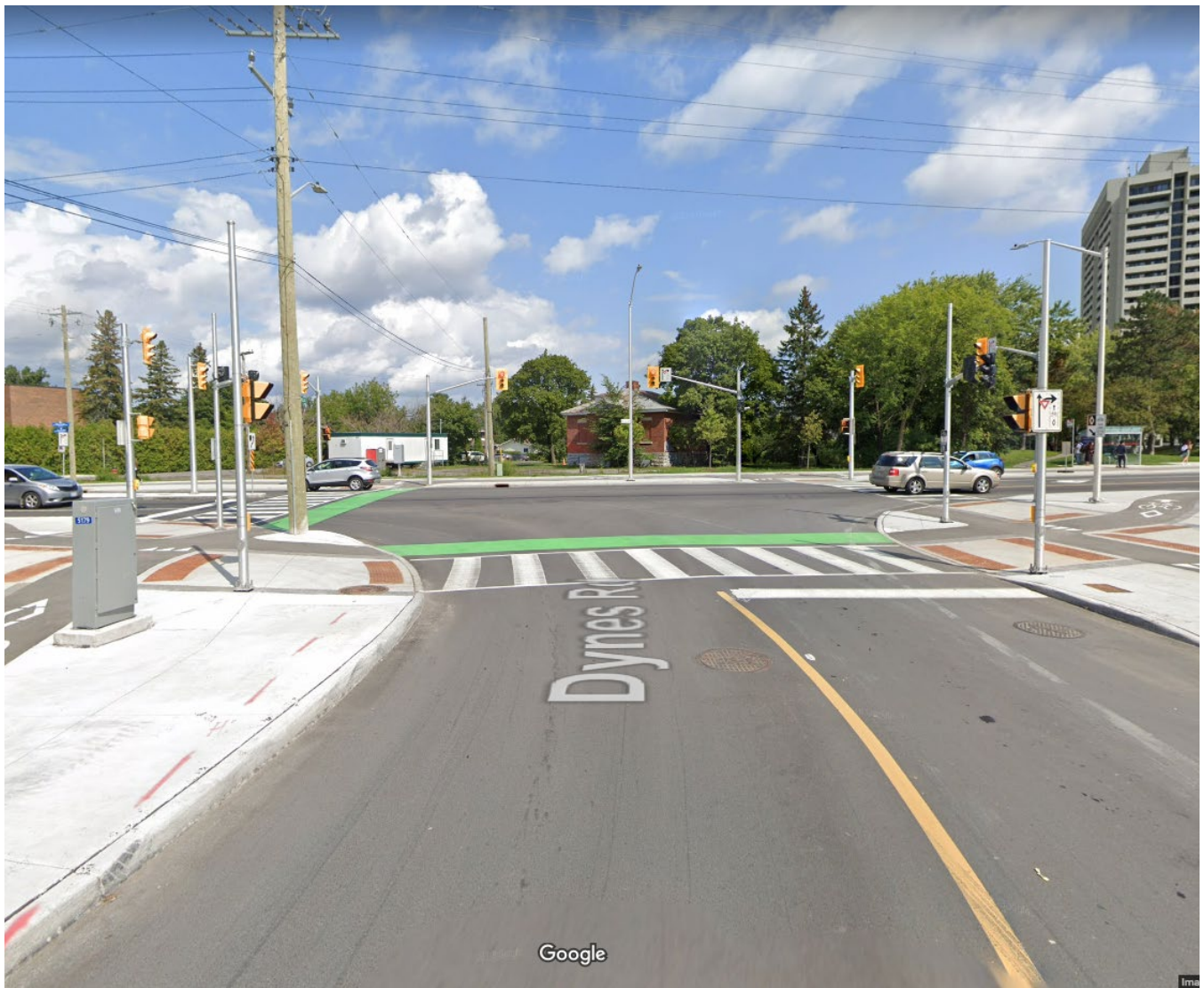
Figure 5: Protected intersection, Dynes Road and Prince of Wales Drive, Ottawa. Image source: Google
