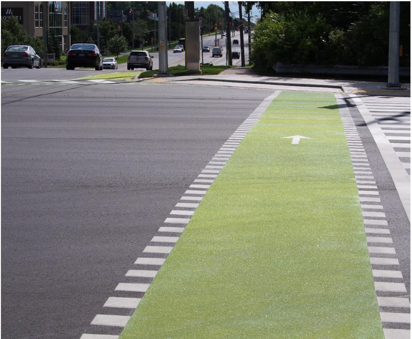
Figure 6: Dedicated intersection crossing at Gordon Street and Stone Road, Guelph. Image source: Morgan Boyco
