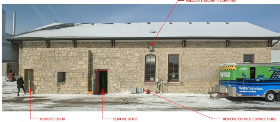
6 SOUTH ELEVATION - PHOTOS 1:100
