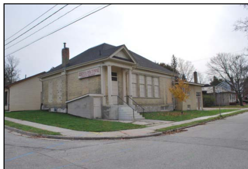
Blocking of window openings should be avoided
