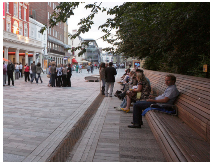
Trench drains delineate between road and boulevard space
