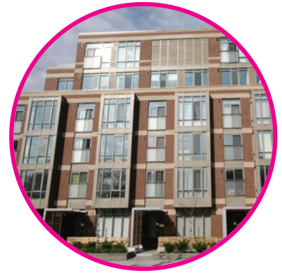
Residential mid-rise building with a landscaped setback and an upper storey stepback
